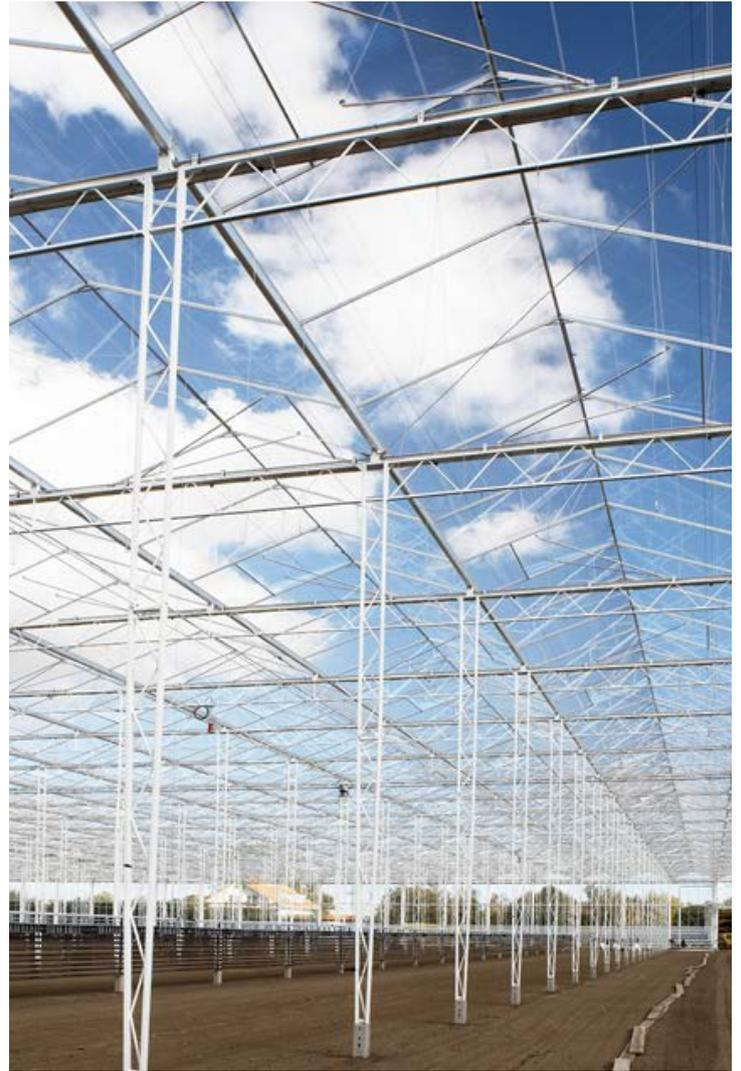
That we are flexible and always looking for ways to optimize our greenhouse systems is proven by the introduction of our Twinlight® column. The Twinlight® column is an open column which consist of less steel and enables the sun to shine through.
