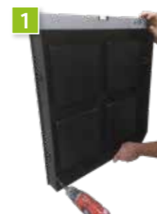
▪ Attach back frame to wall
