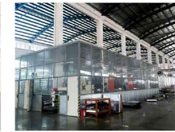
Metal Printing Plant
