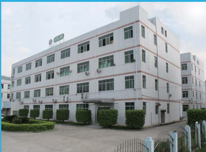
RDI Factory in Shenzhen, China 100,000 sq.ft. manufacturing RDI Technology (ShenZhen) co., Ltd. Tel: +86-755-27333216,27308306.316.326.336 Fax: +86-755-27308799 Website: www.rdichina.com E-mail: sales@rdichina.com
