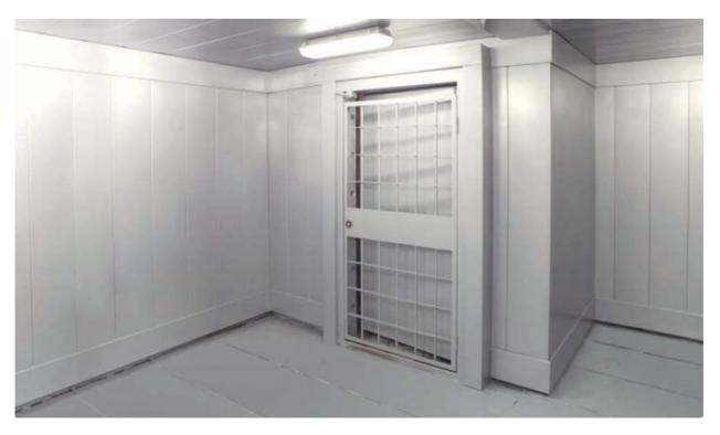
Bank vaults are designed for secure storage valuable things with authorized access. Bank vault consists of two main elements: shell and door block. There are three types of shell: monolithic, modular, combined.
