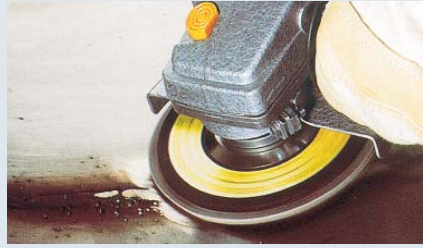
Smoothly flattening welded spot surfaces
