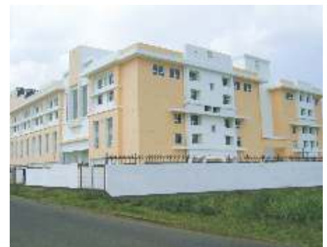
Plant -IV, Gurgaon FCAW, Wear Plates
