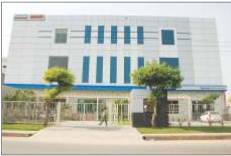
Corporate Office, Gurgaon
