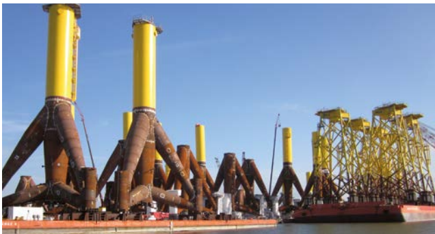
Wind turbine construction
