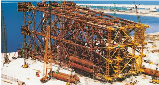
Offshore plant construction: platform
