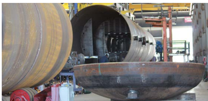
Pressure vessel construction
