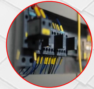
Control Panel Production
